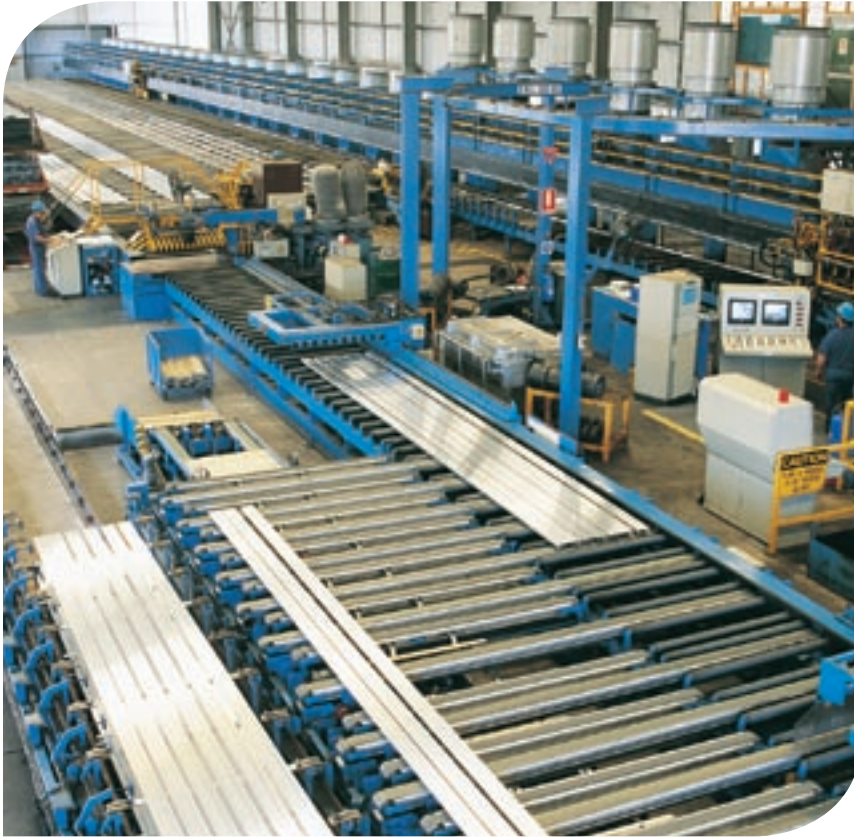
1800 m/t extrusion press and handling system, Brisbane
